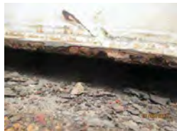
1. Bottom seal damage 2. Under floor plate corrosion
